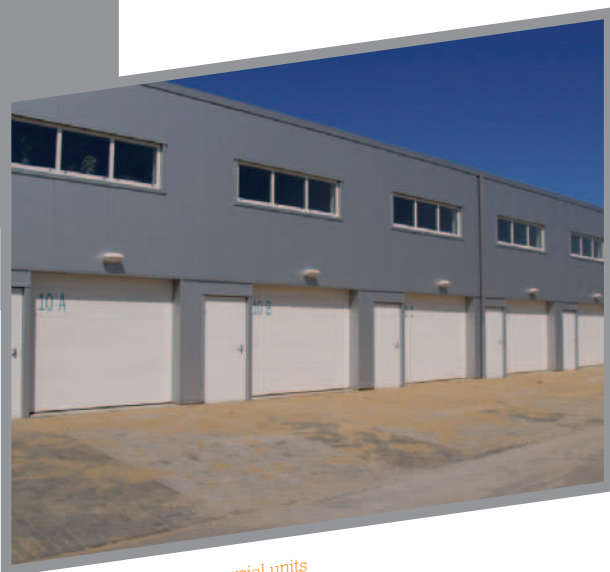
Fire-resistant doors - commercial units
